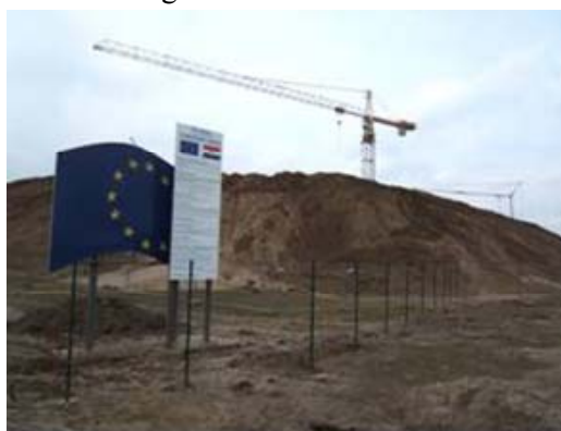
Construction site entrance
