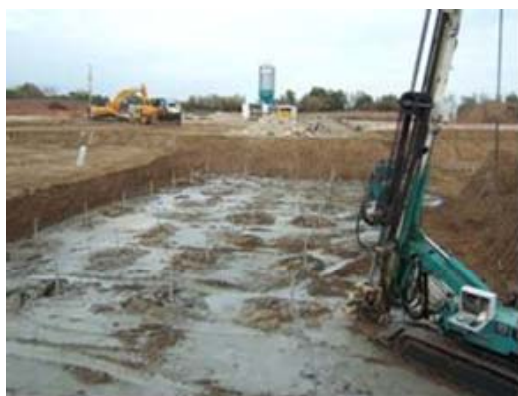
Excavation and piling works
